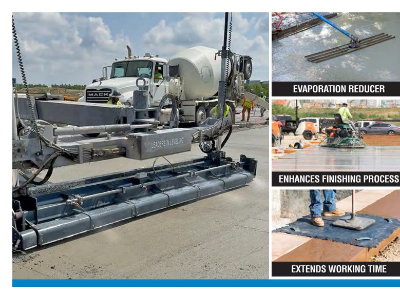
Applied during the floating and troweling process, STAGE 1 combines with calcium hydroxide to form calcium silicate hydrate gels that fill surface pores and capillaries to reduce moisture loss, increase concrete fluidity and extend workability, giving finishers up to an additional 45 minutes of extra finishing time.
