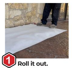
**Roll Out** the Deco-Peel® Blanket on the old acrylic sealer. Trim corners and curves to fit.
