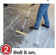
**Roll On** Deco-Peel Liquid Stripper over the blanket until saturated. Allow the liquid to dry. (Usually 2-4 hours).
